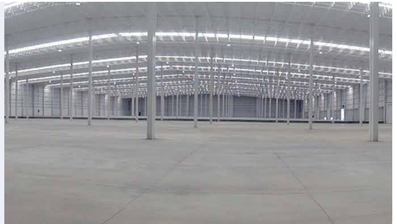
SUNTUF® Skylights Installed
