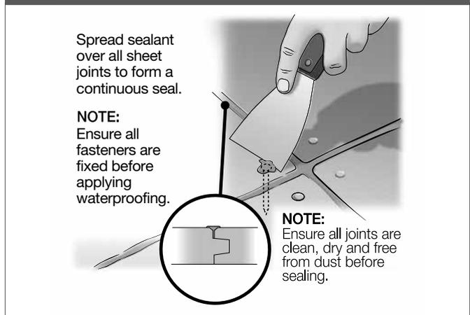
**Note:** Once all sheets are laid for the day, fill tongue and groove, butt joints and fastener heads with sealant. Refer Figure 13.
