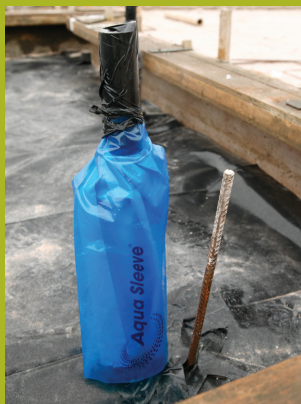
Sleeve between PVC pipe work and concrete.
