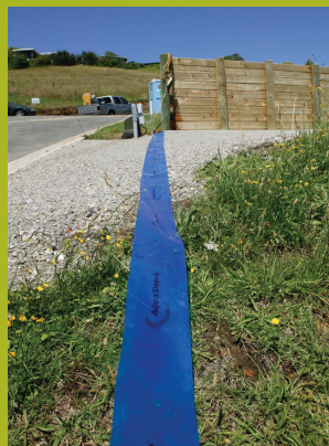
Temporary flexible flume for water control.
