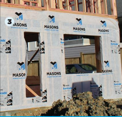
MASONS Barricade™ Building Wrap is a BRANZ appraised wrap that will perform in any area of New Zealand under any cavity-based cladding in up to and including NZS3604 very high wind zones and is weather resistant, durable, and breathable.
