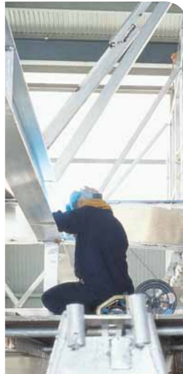
GMA welding of 5383 aluminium with Coregas Argon shielding gas
